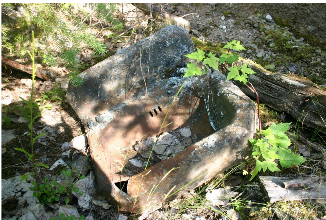
Figure 30. The remains of a metal 2-tap sink found inside the foundation near the SE corner. This is near where a water pipe enters the foundation through a filled-in doorway which leads to a cistern west of the building.
