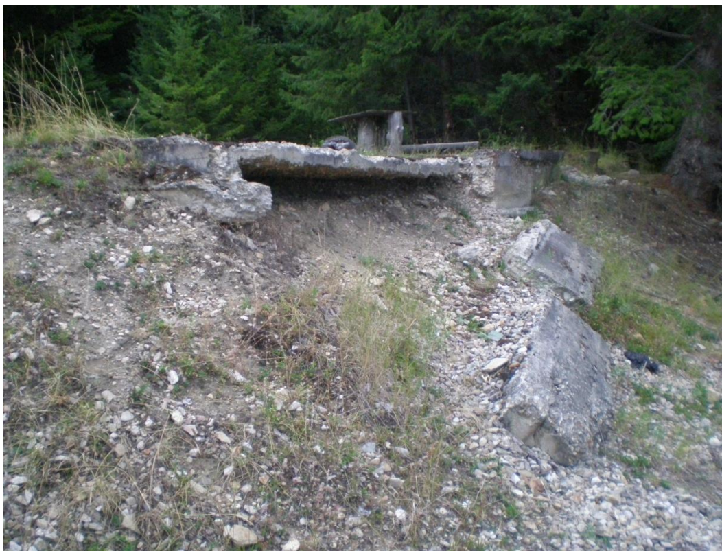
Figure 15. The edge of the concrete slab and retaining wall which were at the front of the City Hotel along Front Street, eroded by the elevated reservoir.
