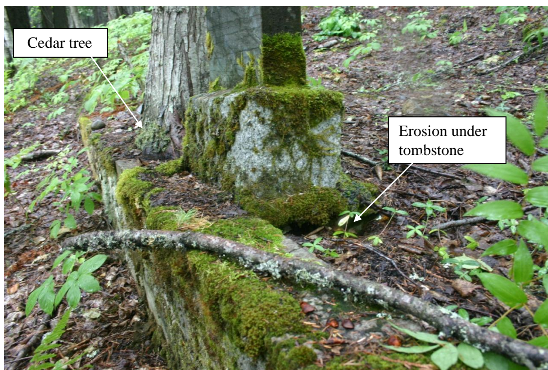
Figure 50. Plot 286 (Johnson), showing undermined tombstone and cedar tree growing over cracked and leaning concrete retaining wall.
