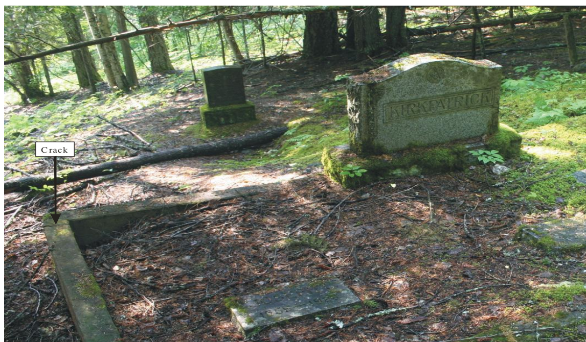
Figure 49. Plot 271a,b,c (Kirkpatrick) showing displacement of soil by erosion inside the retaining wall. The visible crack goes right to the ground and is widening.
