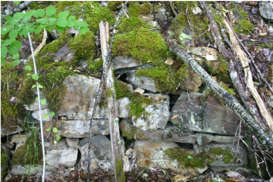
Figure 10. Blocks of local stone were stacked but not cemented to create the wall. A piece of weathered dimensional lumber (3/4" x 3.5" x 4') is leaning against the wall in the centre of the photograph.
