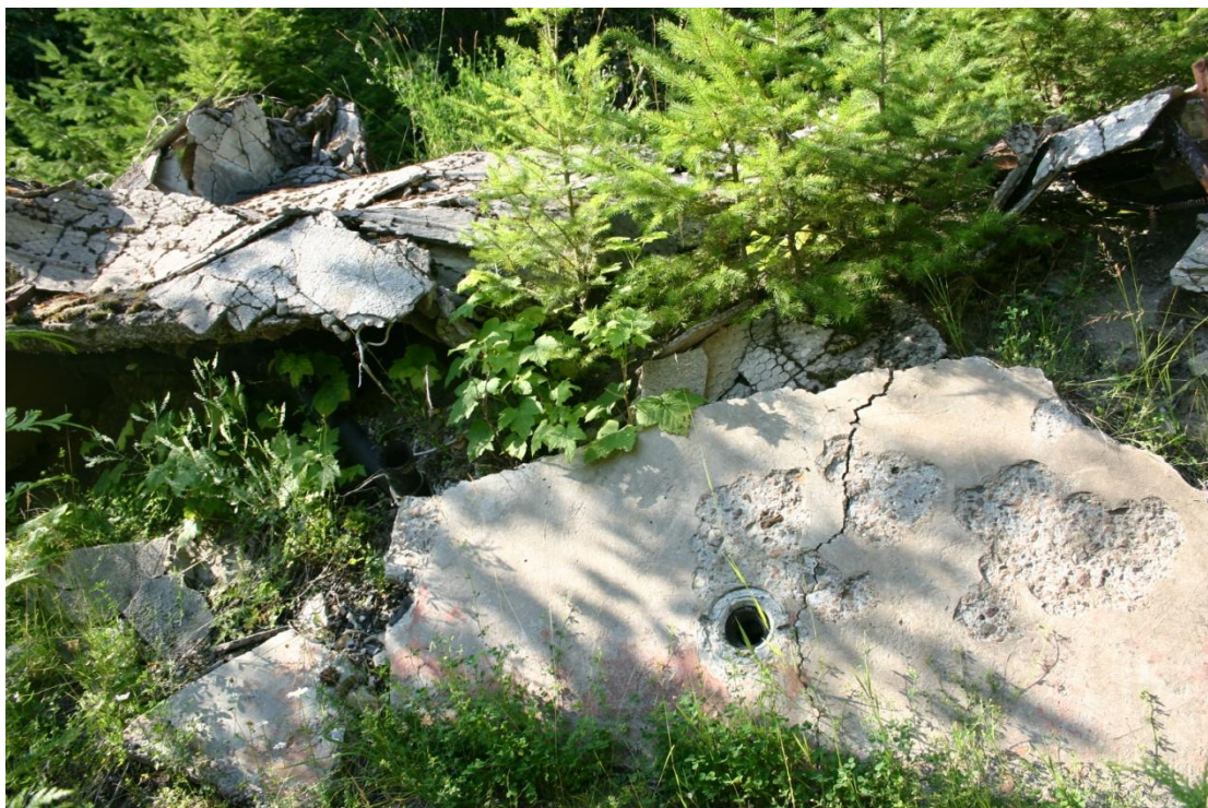
Figure 29. A portion of the collapsed concrete slab at the rear of the building. At least three additional floor drains were plumbed into the 4" slab.
