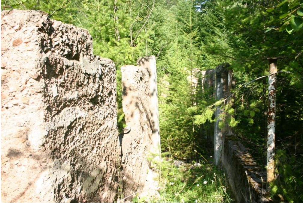
Figure 27. An entrance to the basement at the southwest corner of the school, under where the external stairway to the second floor had been. Variations in the colour and texture of the concrete suggest that this doorway and the low wall to the right were later renovations.
