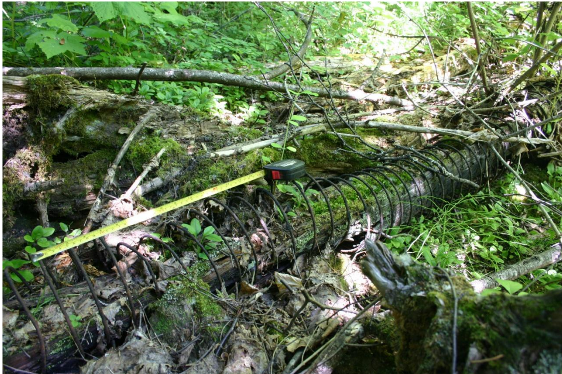
Figure 21. The remains of a wire-wrapped wooden water pipe in Block F.
