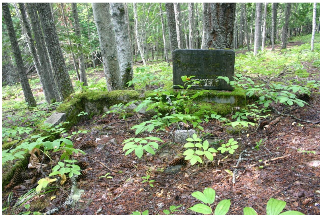
Figure 47. Plot 265 (Bowen). Note severe erosion which has displaced a large amount of soil from inside the retaining wall, and the crack under the stone which is separating from the concrete foundation.
